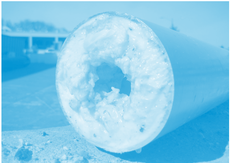
Fats, oils, and grease help to clog municipal sewer pipes creating blockages that can lead to backups and spills.
