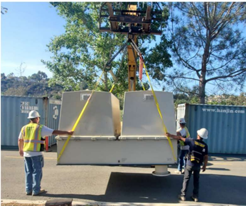
New pressure reducing stations being lowered
