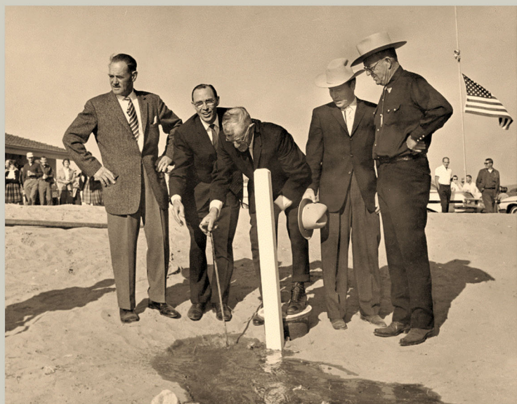
First Board President Alwin "Pop" Wiegand turned on the valve that initiated water flows into OMWD pipelines in 1961
