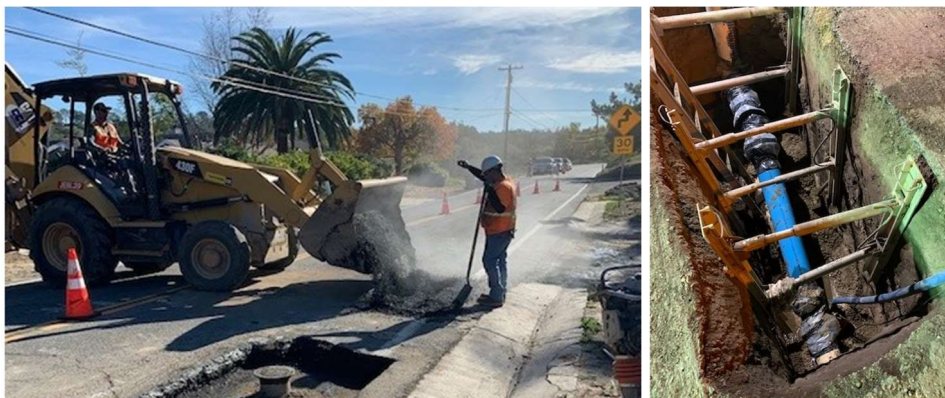
Construction crews installing potable water pipeline along Manchester Avenue
