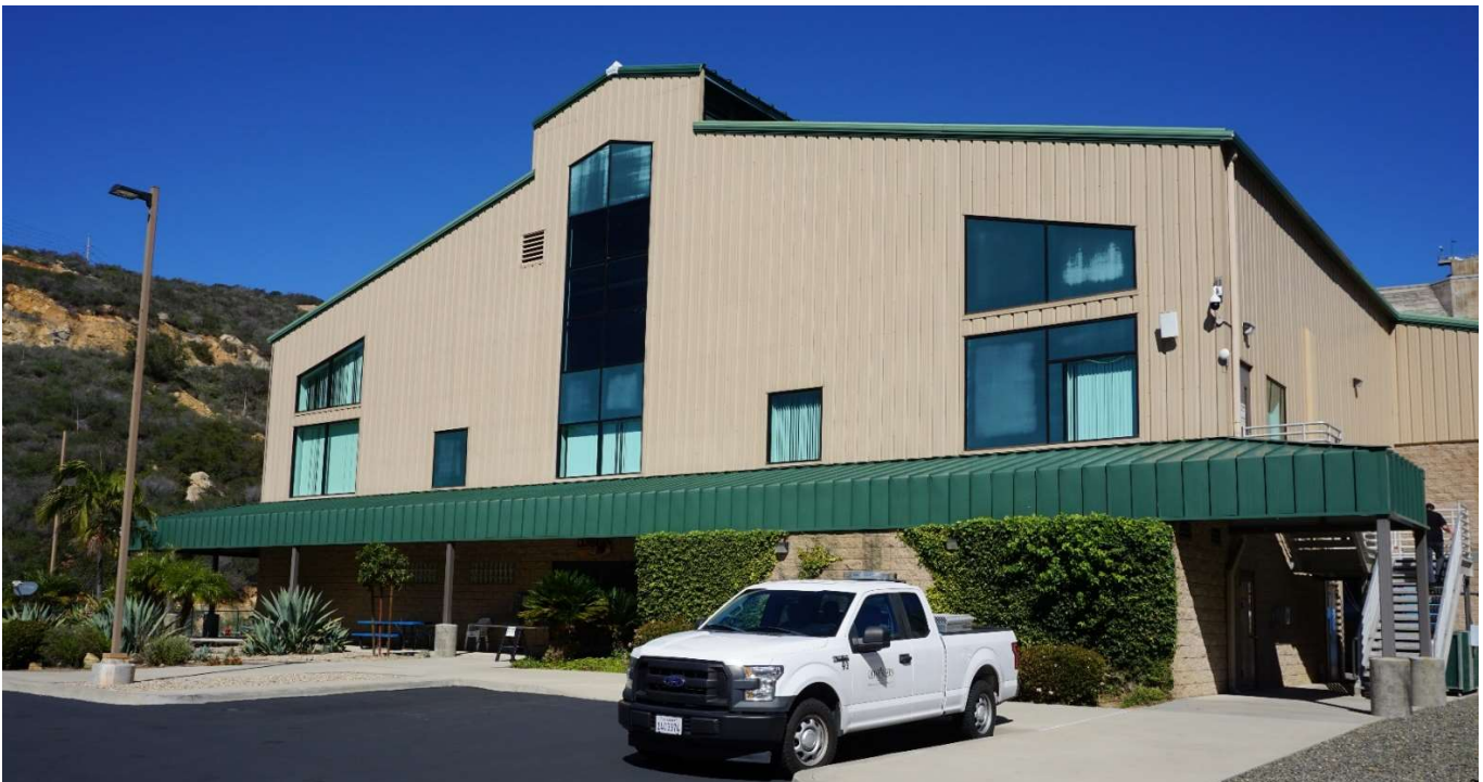
David C. McCollom Water Treatment Plant and the Olivenhain Dam
