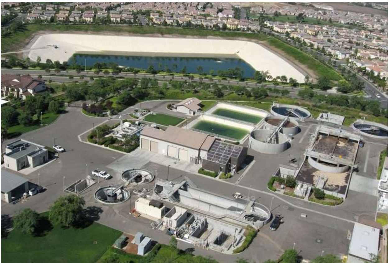
4S Reclamation Facility and Recycled Water Pond
