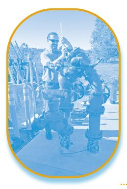
Recently, the Manchester Avenue Recycled Water Pipeline Project was completed in Encinitas. It involved the installation of 7,000 linear feet of recycled water pipeline to provide locally produced recycled water. This project will save over 27 million gallons of drinking water each year by using recycled water instead. By switching from drinking water to recycled water for outdoor irrigation, OMWD is helping to preserve our drinking water supplies for the future.
